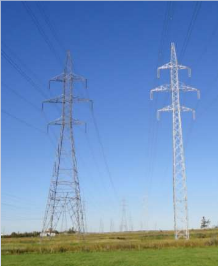
Reduced footprint pylon (selected) next to large footprint pylon
